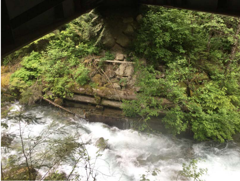
Left Bank Abutment when facing downstream
