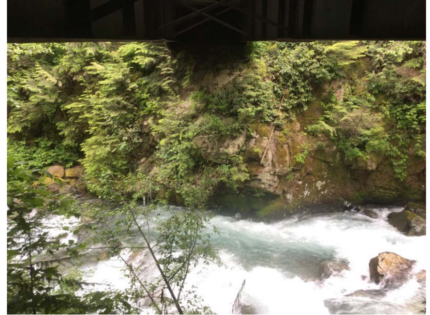
Right Bank Abutment when facing downstream
